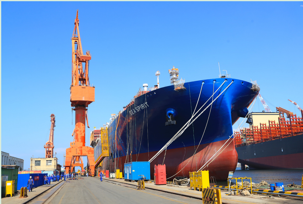
A domestically developed liquefied natural gas (LNG) carrier under construction in Dalian, northeast China's Liaoning Province, on May 15, 2024 (XINHUA)
