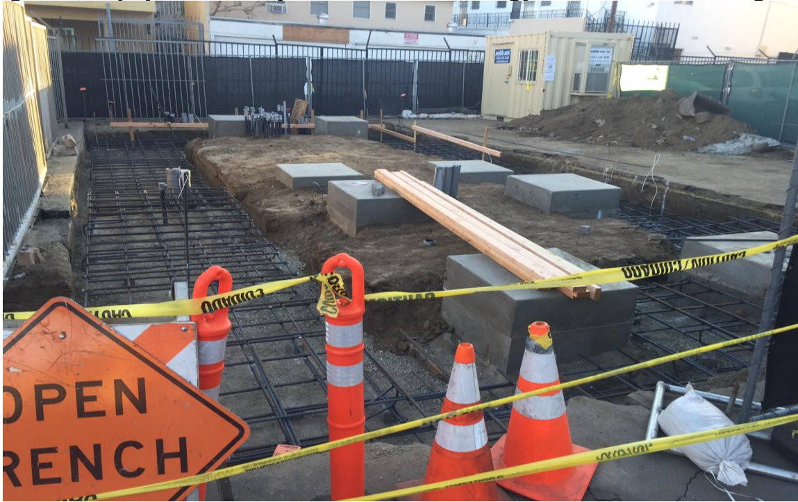
Figure 4: Equipment Pier (Vertical Load Bearing) Foundations In Progress
