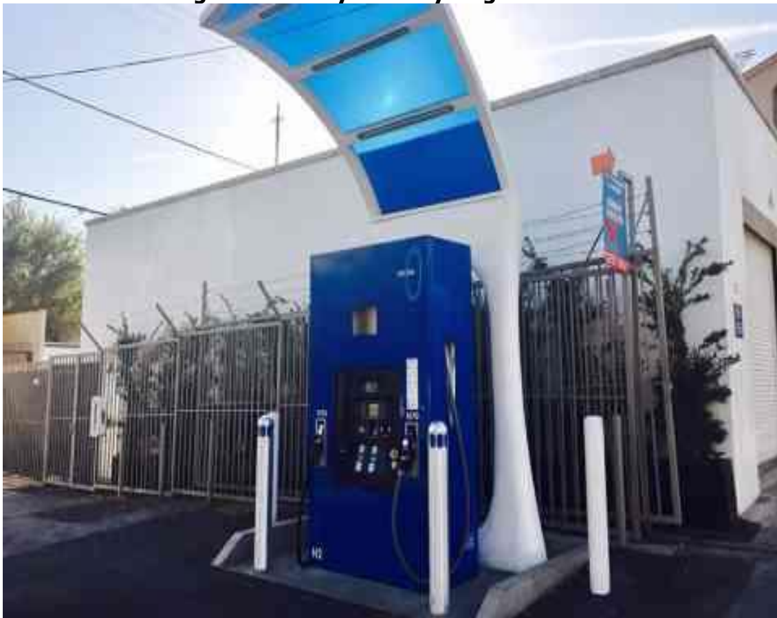
Figure 10: Hollywood Hydrogen Station
