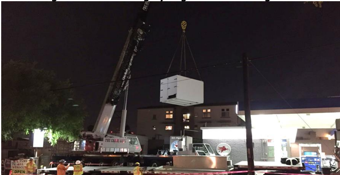
Figure 5: Crane Lifting Hydrogen Ground Storage Unit
